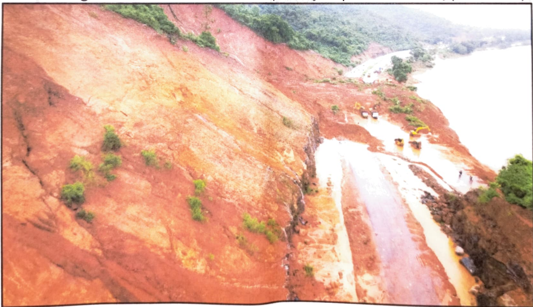
Fig. 5 Transverse cracks on the right flank of the landslide
